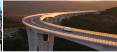
KRINKAL BRIDGE - SLOVENIA
